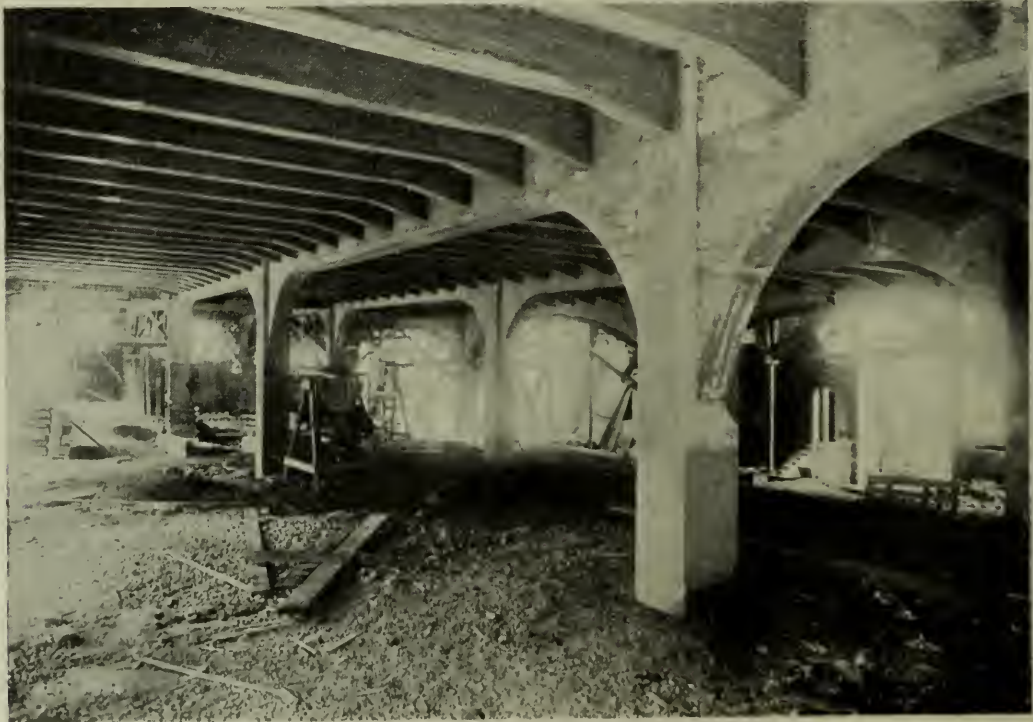
FIG. 3. VIEW BENEATH VIADUCT.
